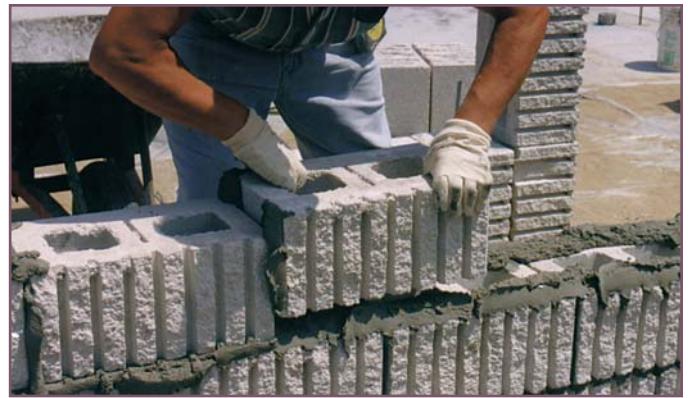
Fig. 1. Use a workable, water-retentive mortar. (IMG13629)
