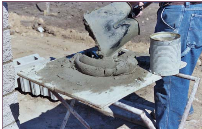
Fig. 2. Retemper mortar as needed to maintain a workable consistency. (IMG13630)
